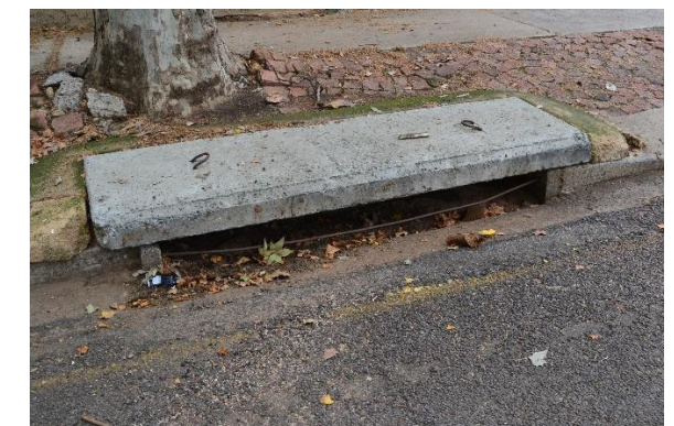
Figure 67: Blocked storm water inlet
