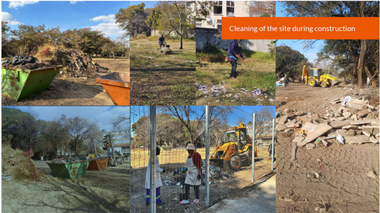
Figure 5 Cleaning of the site during construction
