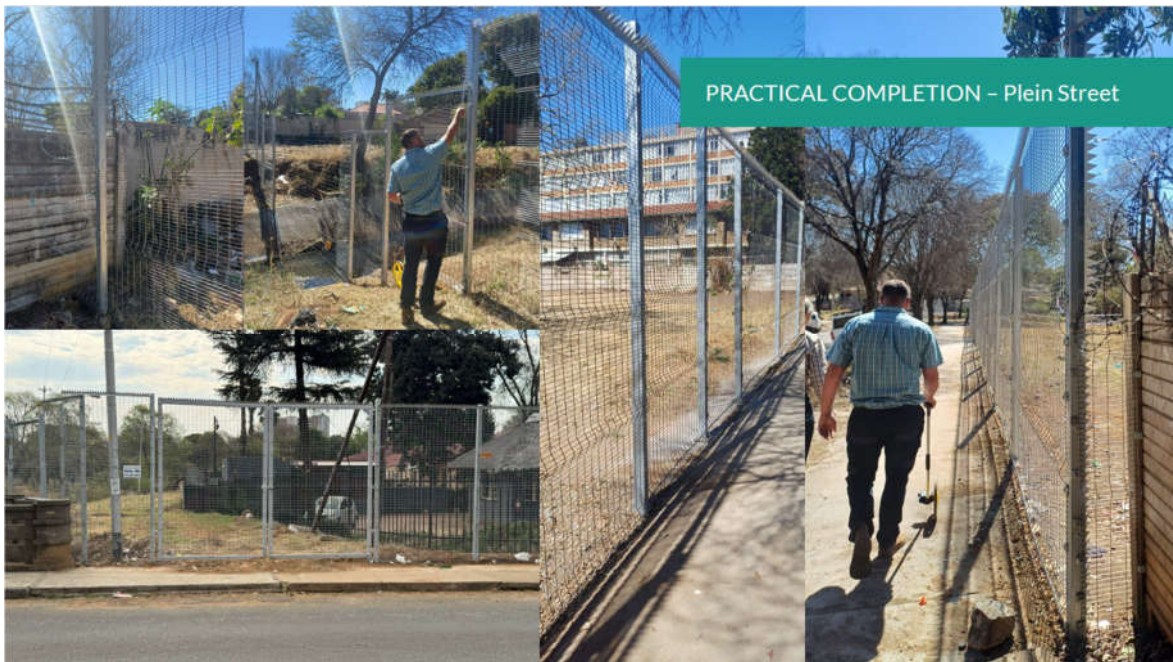
Figure 8 Practical Completion Plein Street
