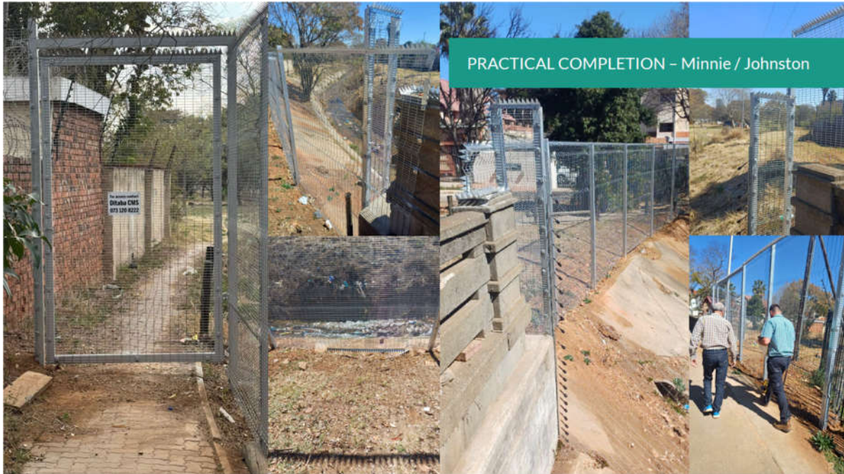
Figure 7 Practical completion of Minnie and Johnston streets
